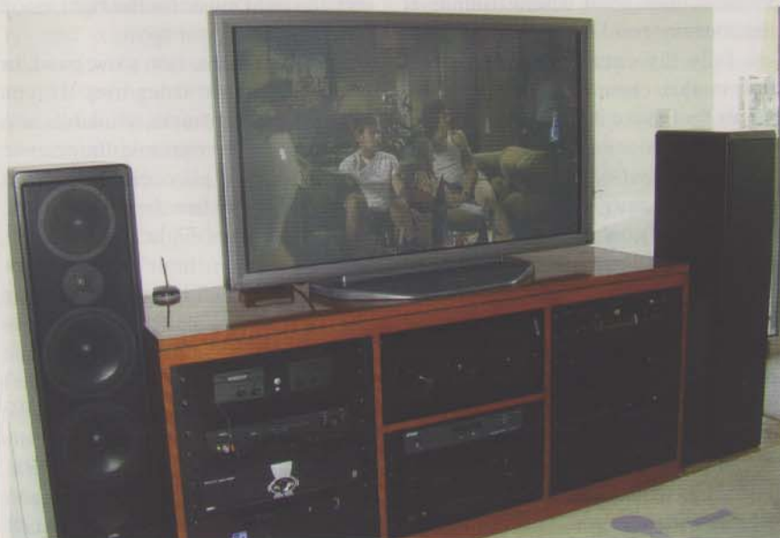
This consumer installation features an unusual custom cabinet, designed so that electronics elements could be rack-mounted and the center-channel speaker could slip into the allotted area. The floorstanding speakers are part of the Canton Ergo series
