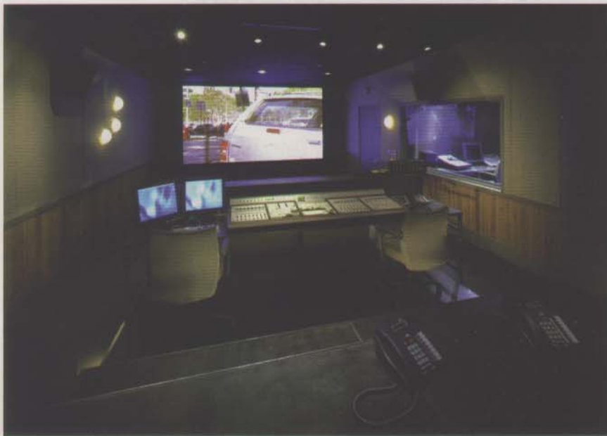
The Dig It Audio Productions studio in New York City. Here, Rothstein designed both the 7.1-channel audio and video monitoring systems. The installation represents one of the earliest "multi-curve" audio systems, enabling engineers to switch seamlessly between cinema sound's Academy (classic theater) Curve and Dolby-X (new theater) Curve
